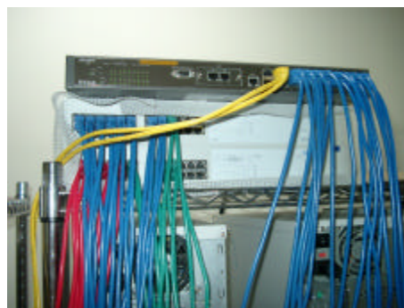
Figure 7: Apply channel bonding technique by using three switches
